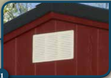
1 8x16 aluminum vents standard on all buildings
