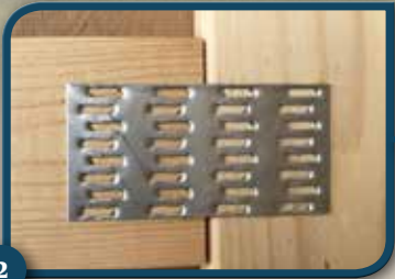
2 2x4 truss plates standard on all doors and trusses
