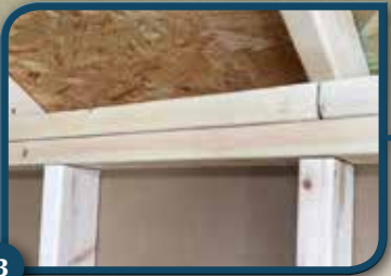
3 16" on center wall studs and 2x8 top plate
